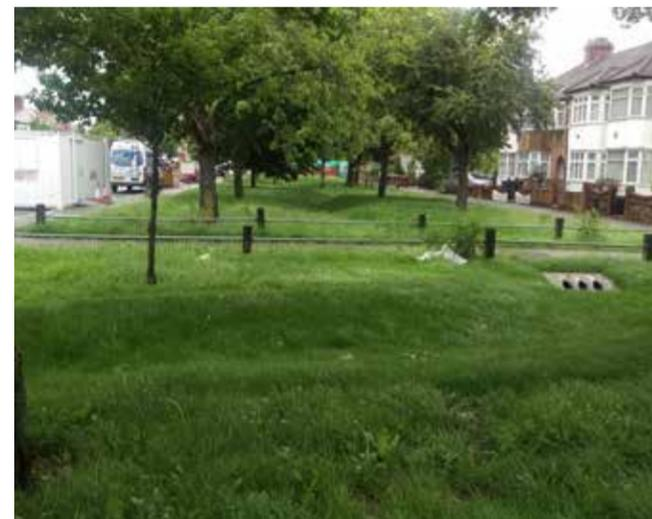
Surface collection in channels, gutters and permeable pavements, or as sheet flow onto grass surfaces, keeps runoff at or near the surface, enabling cost-effective and visually legible design.
