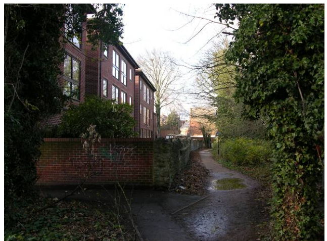
Looking north along stretch of medieval Rewley Abbey Wall fronting onto the Castle Mill Stream
