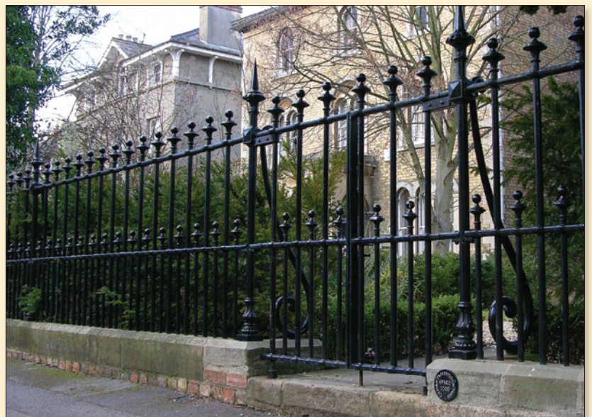
Restored railings in Park Town, Oxford
