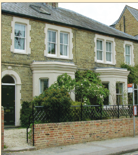
Left, renovated wall and reinstated railings fronting Kingston Road
