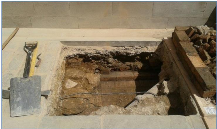
Above: Investigation of the ground prior to the construction of foundation pads for the new bin store. Re-used column base bottom left.
