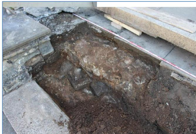
*Above: Opening up work to investigate the character of the steps in Tom Quad—the top 'step' returns north and appears to be bonded with the buttress. It is possible that some of this fabric is Wolsey's original build, adapted in 1841 and again in the early 1870s. Photograph by Graham Keevill.*
