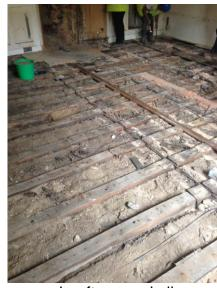
that the timber has previously been used as a pegged rafter or similar, however, the joists did not display any other signs of reuse such as nail holes, other than those obviously associated with the floorboards, and may therefore be related to previous timber treatment.
