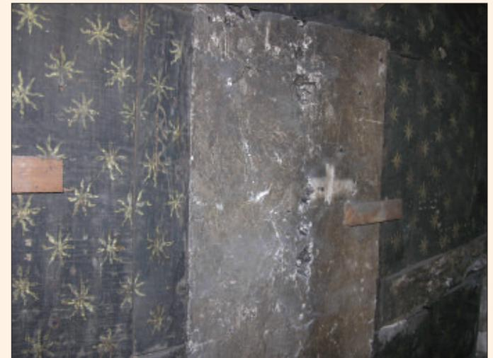
**Fig. 30** Painted panelling and a door from a previously unknown 17th or early 18th century student study exposed at Brasenose College during building work in 2010.
