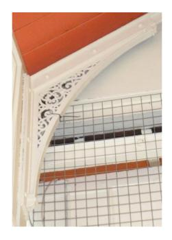
Fig 15: View of cast iron roof in the Covered Market.
