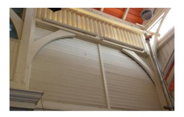
Fig 25: View of horizontal timber louvers along the east wall of avenue 4.
