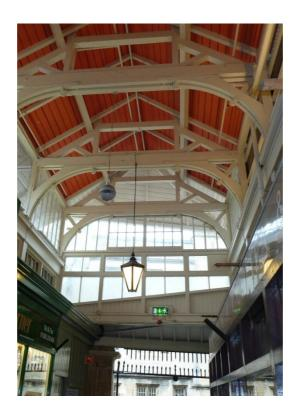
Fig 24: View of queen post roof with braces
