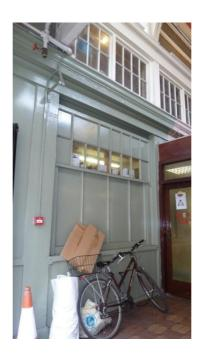
Fig 26: View of large timber sash with horns
