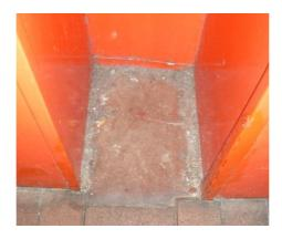
Fig 23: View of terracotta floor tile under the shop front of No 98.
