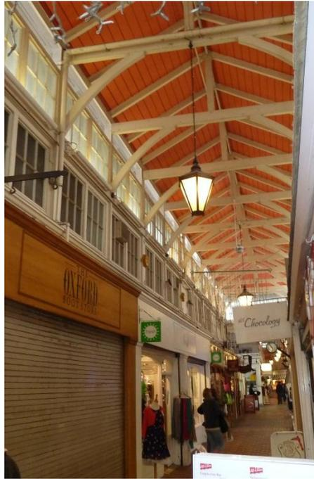
**Fig 21: View of king post roof along avenue 1 looking north**
