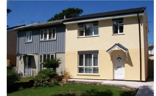
Image: Low Carbon Hub. Houses before (left) and after (right) deep retrofit measures. External wall insulation among one of many retrofit measures applied.
