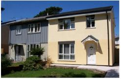
Image: Low Carbon Hub. Houses before (left) and after (right) deep retrofit measures. External wall insulation among one of many retrofit measures applied.
