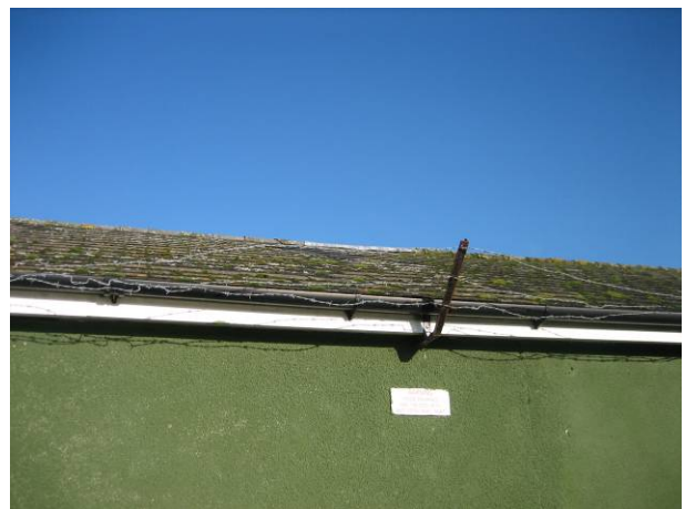
Figure L: Loose lead flashing along ridge at north-west end of roof
