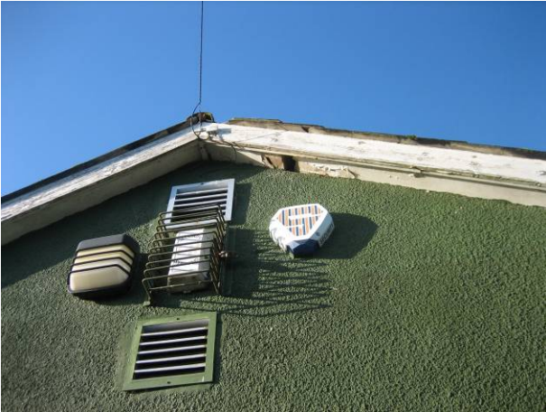
Figure I: Hole in soffit board, also with bird droppings
