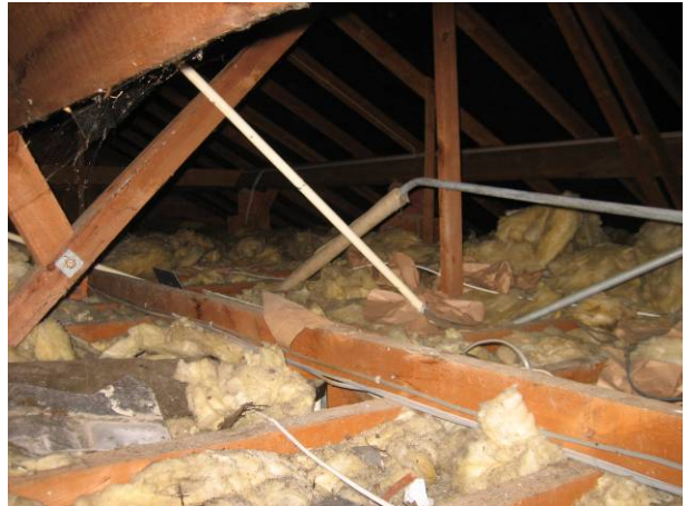
Figure D: Attic floor showing pipes and insulation
