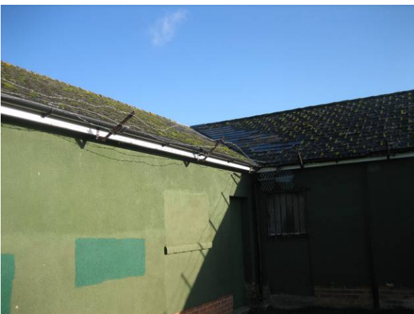
Figure K: Lead flashing at roof join
