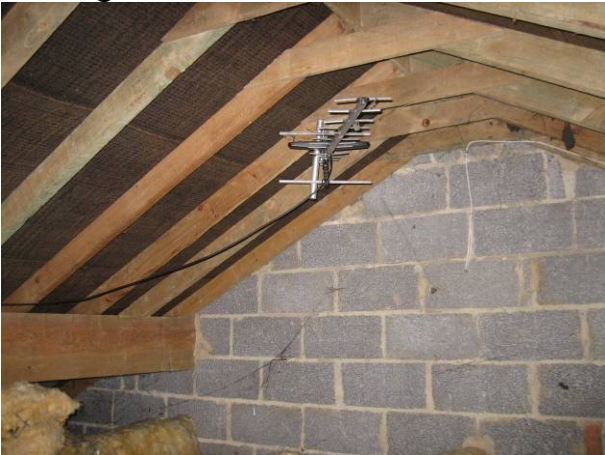
Figure C: Structure of roof from inside showing beams and internal wall
