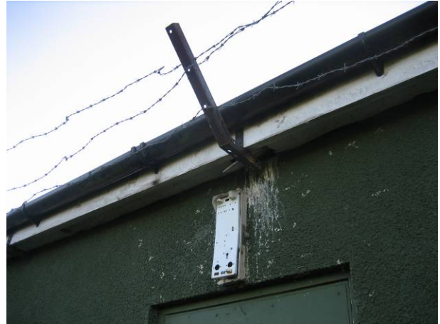
Figure J: Hole in soffit board with old bird nesting material present
