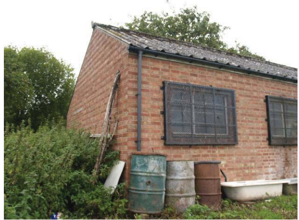
Figure D: Allotment building – detail of flush barge boarding
