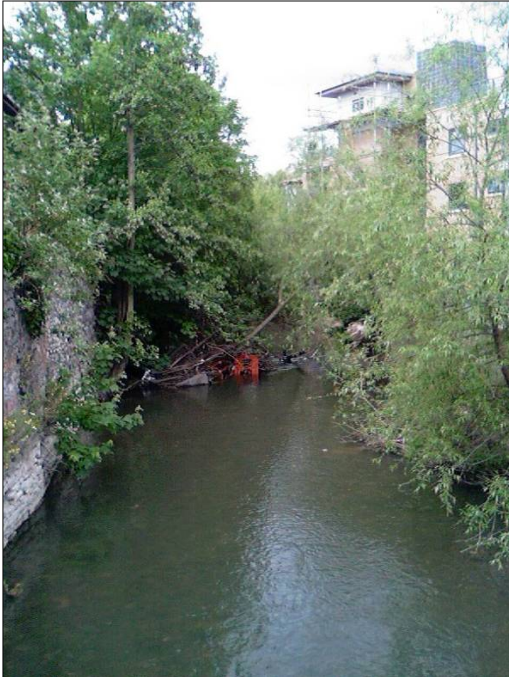
Figure 2: In Channel Vegetation and Debris Material in Wareham Stream
