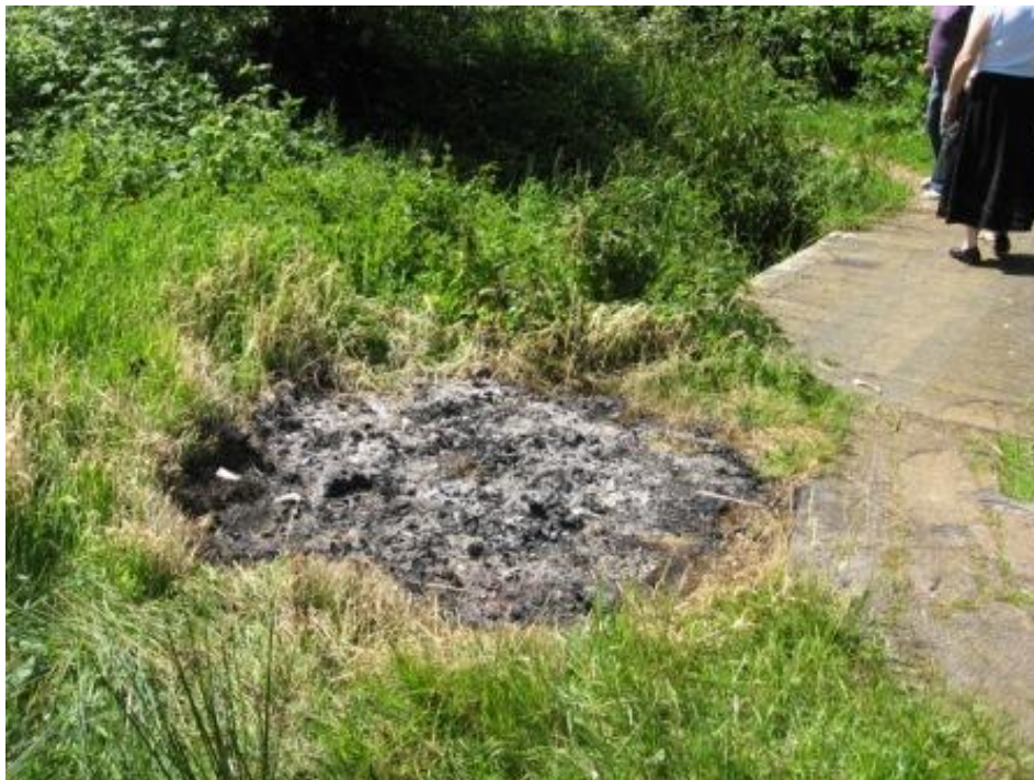
Arson damage actually on the North Fen SSSI, May 2007
