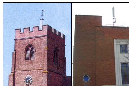
Photo 2: Listed buildings: (a) Antennas disguised as weathervane (b) Poorly sited antennas
