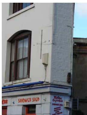
Photo 1: Example of a microcell antenna which could be classed as 'de minimis'
