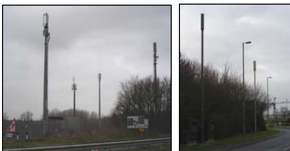
Photo 6 (a) & (b): Multiple masts can cause unacceptable clutter (examples in Oxford area)
