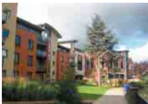
4. Articulation of massing and roof line presents a varied silhouette to the sky
