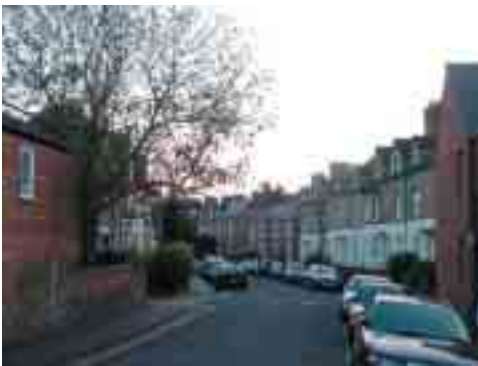
2. 'Big box' inset from the corner allowing buildings more active frontages to face the side street
