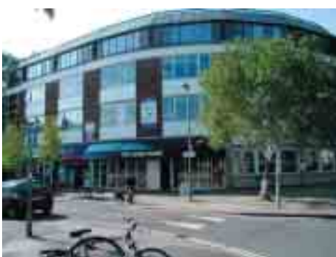
2. A four storey building to the main street and return frontage to the side street
