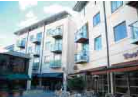
2. Vertical emphasis through alignment of windows and balconies and downpipes
