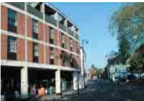
3. Bays and storey heights expressed to give both vertical and horizontal rhythm
