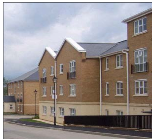
Affordable housing at Elizabeth Jennings Way
