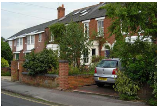
Front garden parking should be integrated into the street scene (Grandpont, Oxford)
